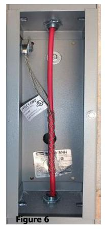
8. Vertical Cable Supports – (Figure 6). Vertical runs beyond the maximum distances described in Section 7 require the cables to be supported using an AMTEC stainless steel wire mesh support grip within a vertical enclosure.
